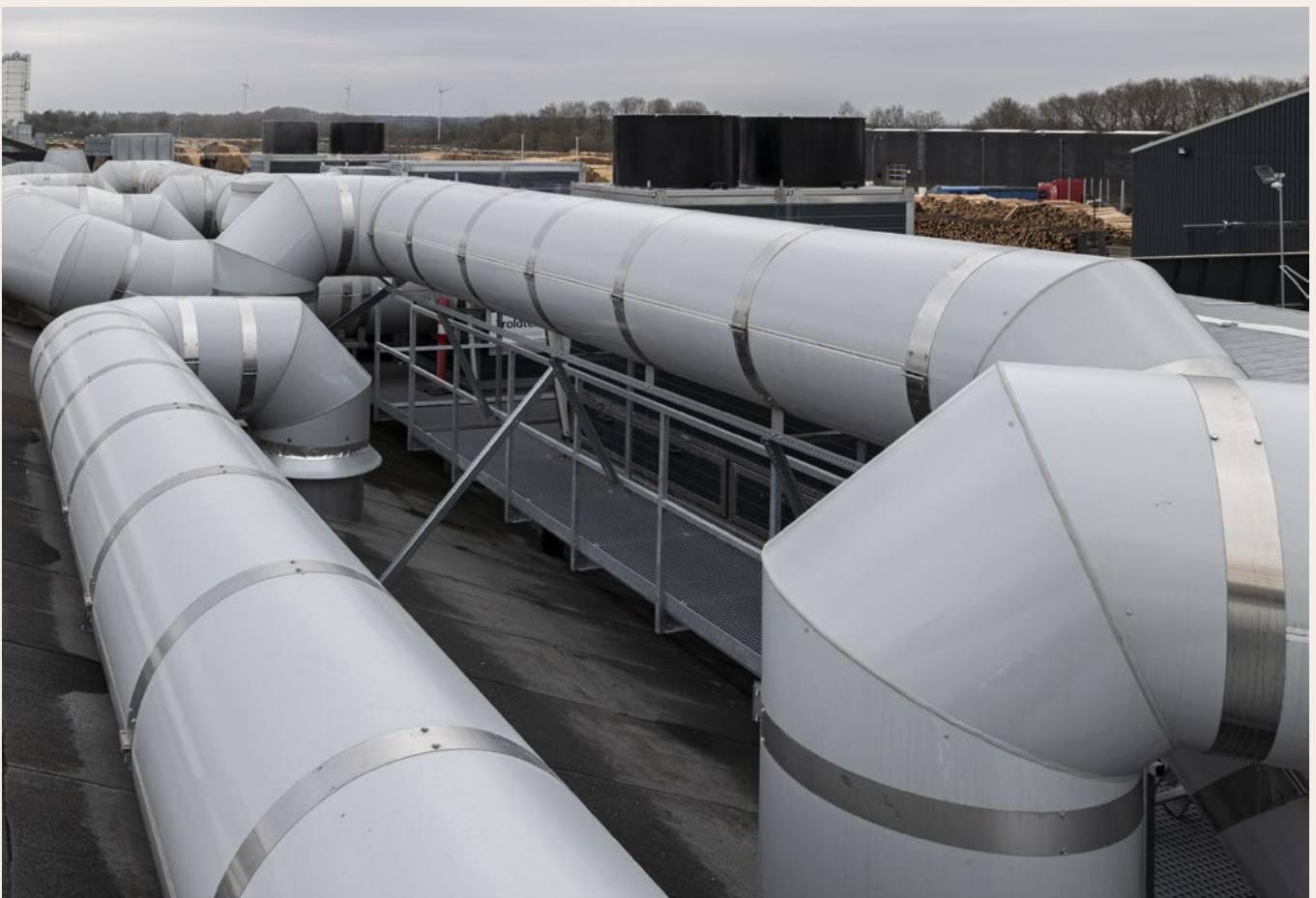
Troldekt has expanded a pilot project on heat recovery in our drying process by installing an additional seven heat exchangers. The additional heat exchangers have the potential to reduce our fuel consumption by around 20%. Read more on page 28..
